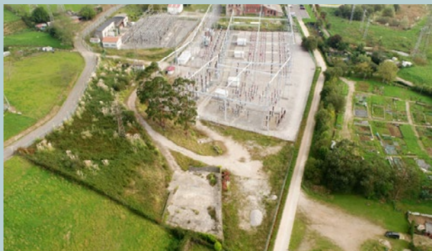
Aerial picture of the aspect of the substation
